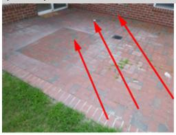
The patio surface is sloped to encourage storm drainage back toward the home. Drainage toward the foundation and framing areas can result in damage to the siding, doors, adjacent structural components, and allow water to enter the home resulting in undesirable conditions (see rear sliding door comment). A licensed general contractor should be consulted for further evaluation, to determine the extent of the concern, and make necessary repairs.
