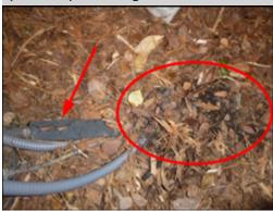
The large line of the AC refrigerant line set that connects the outside compressor unit to the interior air handler is required to be insulated to reduce condensation and associated water damage. The AC line insulation is missing/damaged and is buried under the landscaping at the exterior of the home. A HVAC contractor should be consulted for a complete evaluation and repair of the system to ensure reliable and proper operation of the HVAC system.
