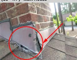
The flashings system around the chimney is damaged/heavily caulked. A licensed roofing contractor should be consulted for evaluation to determine the source of the leak, the extent of the damage, and repair as needed.
