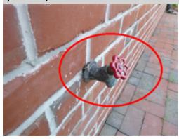
The exterior faucet located at the rear of the home is not a frost free or anti siphon fixture. Although not required when this home was built, the anti-siphon faucet prevents back flow related to pressure drops to prevent contamination of the water supply and piping systems. The buyer should consider upgrading the exterior faucets.
