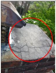
The mortar crown is deteriorated and cracked. When the mortar crown is damaged water can enter between the chimney body and the flue liner resulting in leaks and deterioration. A masonry contractor should be consulted for a complete evaluation of the chimney, the flue liner and the masonry crown and to make necessary repairs.
