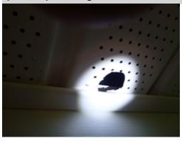
The secondary overflow which is connect to the condensate pan in the attic is not properly aligned to discharge out of the hole in the soffit vents. This cause two issues: the first is if the secondary is needed, the condensate will be draining into the attic and not out of the home and second, the hole has allowed a penetration for insects/animals to enter the attic. A licensed HVAC contractor should be consulted to repair the situation.
