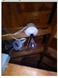
The light fixture in the attic by the attic ventilation fan was not functional when tested. This could indicate a defective bulb or other more serious problem such as faulty wiring or a defective fixture. A licensed electrical contractor should be consulted for further evaluation and repair.
