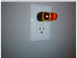
The GFCI receptacle for the master bathroom by the toilet did not operate properly when tested. The GFCI is an important safety feature that should be kept functional to reduce shock hazards. A licensed electrical contractor should be consulted for repair.
