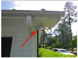
The light fixture by the front left side of the home was not fully functional when tested. One of the lights on the fixture would not turn on. This could indicate a defective bulb or other more serious problem such as faulty wiring or a defective fixture. A licensed electrical contractor should be consulted for further evaluation and repair.
