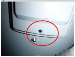
The maintenance cover panel on the hot water heater is missing screw. This could result in damage to the controls inside and also anyone who is trying to gain access. The screw should be replaced to ensure safety.
