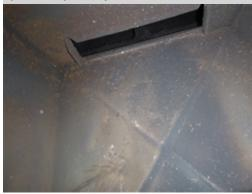
From the fireplace insert opening, heavy build of creosote was noted. Creosote build-up can result in improper function of the fireplace and high potential for fire. A chimney sweep and general contractors should be consulted for a complete evaluation of the chimney and to make necessary repairs to ensure that the chimney is safe and functional.
