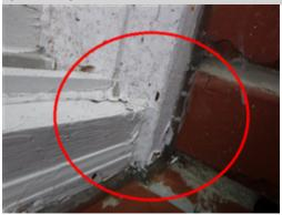
The garage windows have visible wood filler repairs. Wood filler is used as a temporary repair when wood decay is present. Decay in the windows can result in leaking and water penetration and should be repaired as soon as possible. Since wood filler repairs have a limited life and depend on the complete removal of all decay, the repairs need further evaluation. The homeowner should be asked for disclosure related to the age/extent of the repair and any history of leaks.
