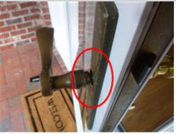
The storm door at the front of the home is in need of repair , the doors handle was loose. Technically a storm door is not covered by the home inspection SOP, however, when the handle is loose it creates a safety issue. A repair specialist should be consulted for repair or replacement.
