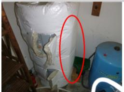
The Temperature Pressure Relief Valve (TPRV) for the water heater is a safety device to prevent the unit from exploding in case of a malfunction. The TPRV has been covered by the insulation applied around the tank. This prevents visual evidence that the TPR valve has released. A licensed plumber should be consulted to reapply the insulation around the tank where the TPRV is on the outside of the insulation.
