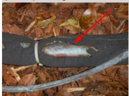
The large line of the AC refrigerant line set that connects the outside compressor unit to the interior air handler is required to be insulated to reduce condensation and associated water damage. The AC line insulation is missing/damaged at the exterior of the home. A HVAC contractor should be consulted for a complete evaluation and repair of the system to ensure reliable and proper operation of the HVAC system.
