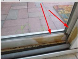
The stains on the door frame/door wall for the sliding glass door to the patio indicate that the door leaks at the door area. Water penetration can result in hidden damage and undesirable conditions. A general repair specialist or licensed general contractor should be consulted for a complete evaluation to determine the source of the leak, to locate any related damage, and repair as needed.
