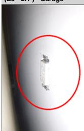
The receptacle in the garage (GFCI) has a missing cover plate. A missing receptacle cover plate could result in increased shock and fire hazards. A general handyman should be consulted to install a new cover plate.
