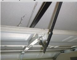
The garage door on the left side needs adjustment and repair. The door did not stop/reverse when the path was interrupted. A garage door installation company or a licensed general contractor should be consulted for evaluation and repair to ensure that the door operates safely and properly.
