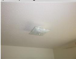
The light fixture to the right side inside the garage was not functional when tested. This could indicate a defective bulb or other more serious problem such as faulty wiring or a defective fixture. A licensed electrical contractor should be consulted for further evaluation and repair.
