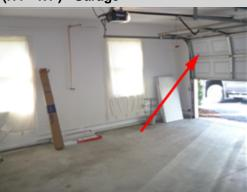
The right side garage door needs adjustment and repair. The door lift motor was very loud and strained as it raised and lowered the door. A garage door installation company or a licensed general contractor should be consulted for evaluation and repair to ensure that the door operates safely and properly.
