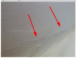
Soft spots and repairs on the walls above the whirlpool indicate a history of condensation. A licensed general contractor should be consulted to review the conditions and make necessary repairs.
