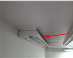
The light fixture under the cabinet by the sink in the kitchen was not functional when tested. This could indicate a defective bulb or other more serious problem, further evaluation is needed. A licensed electrical contractor should be consulted for further evaluation and repair.
