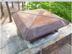
The chimney cap is rusted. The corrosion could indicate the age of the cap or that the cap is not properly installed. If the cap is not functioning properly it could direct drainage or moisture into the flue or roof area. A masonry contractor should be consulted for a complete evaluation of the chimney, the flue liner and the masonry crown and to make necessary repairs.
