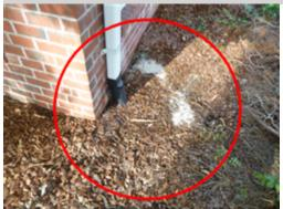
Evidence on the bedding and ground areas indicates that the roof drainage has been overflowing the gutter trays a the right rear of the home. Direct drainage to the foundation and cladding from the gutter system can result in water penetration into the foundation area and foundation deterioration. A licensed general contractor should be consulted for a complete evaluation of the gutter system to reduce overflow and to make necessary repairs.
