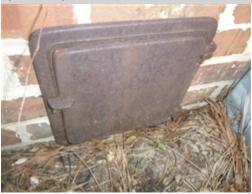
The fireplace cleanout door is damaged and in need of repair/replacement. The cleanout door prevents active or hot embers from entering unprotected areas. The chimney needs a complete evaluation and invasive inspection prior to use. A chimney sweep and general contractors should be consulted for a complete evaluation of the chimney and to make necessary repairs to ensure that the chimney is safe and functional.
