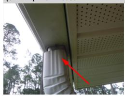
The downspout at the front of the home is not securely connected to the gutter. This can result in improper drainage and increases the opportunity for the downspout to become disconnected from the gutter. A licensed roofing or gutter contractor should be consulted to repair.
